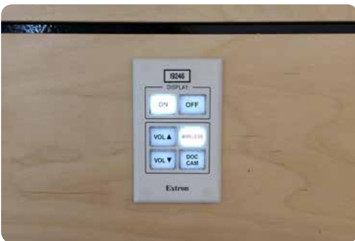
The Extron 6 button control panel simplifies operation in the new POD classrooms.
