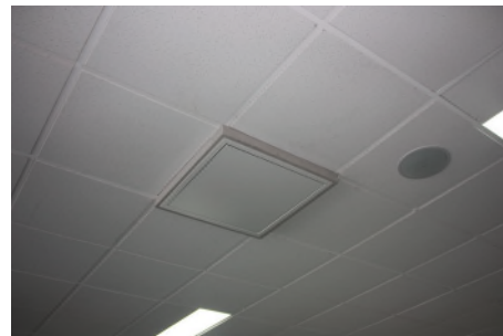
CCCC – Projector fully recessed into ceiling
