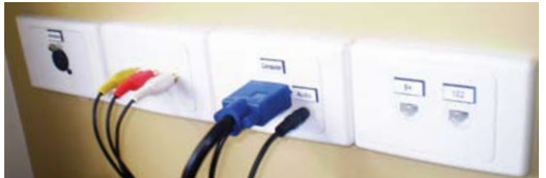
ABOVE: Connection points, including microphone socket and VGA and stereo audio input FAR LEFT: Joey Micro along with speaker volume control LEFT: EPSON EMP-83 is projected onto this manual screen
