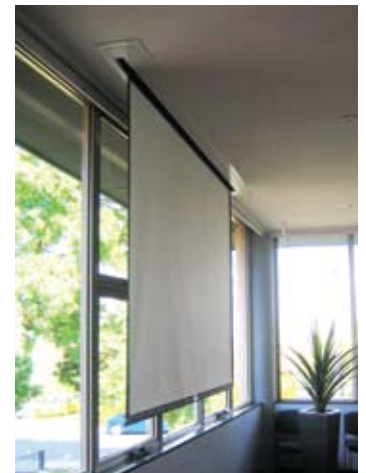
LEFT: Flipper mounting bracket hiding the projector up in the ceiling when not in use
