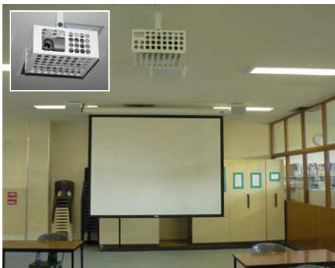
Above: Control Panel and computer inputs are kept safe in a security cabinet. Left: Motorized screen is ceiling mounted ensuring screen is safely stored when not in use Inset: Epson projector mounted to ceiling using security cage.
