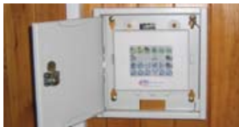
TOP: Wall box houses the Joey Lite control panel, keeping it protected.
