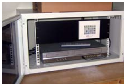
BOTTOM RIGHT: AV wall cabinet housing the DVD/VCR combo player, along with a Joey Lite control panel that enables teachers easy projector operation at the touch of a button.
