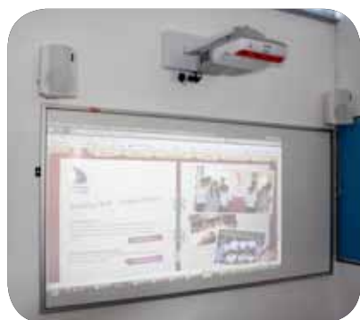
ABOVE: An Epson EB-450We Ultra Short Throw Projector and 2Touch Interactive Whiteboard installed in Glenroy College's conference room
